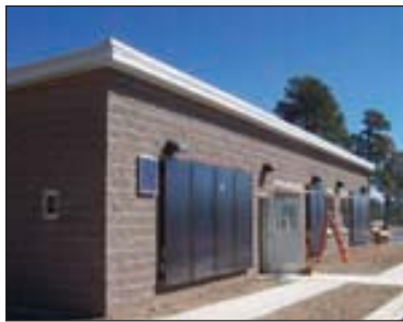
Figure 3. South face of Eco Station uses PV panel for solar glycol pump (30-watt rating) and Viessmann solar heat collectors with shipping covers removed.
